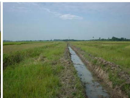
After renovation of canal
