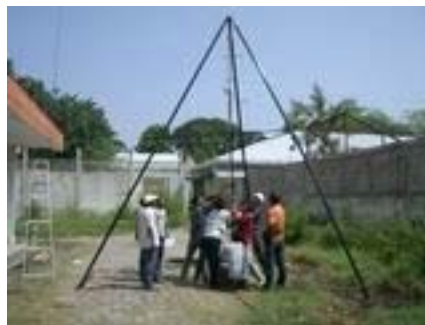
Standard Penetration Test (Blowing)
