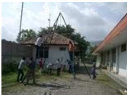
Standard Penetration Test (Preparing Tripod)
