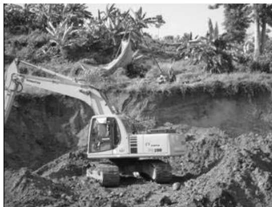
Gambar E-3.3 Tambang Material Tanah ( Borrow Soil )
