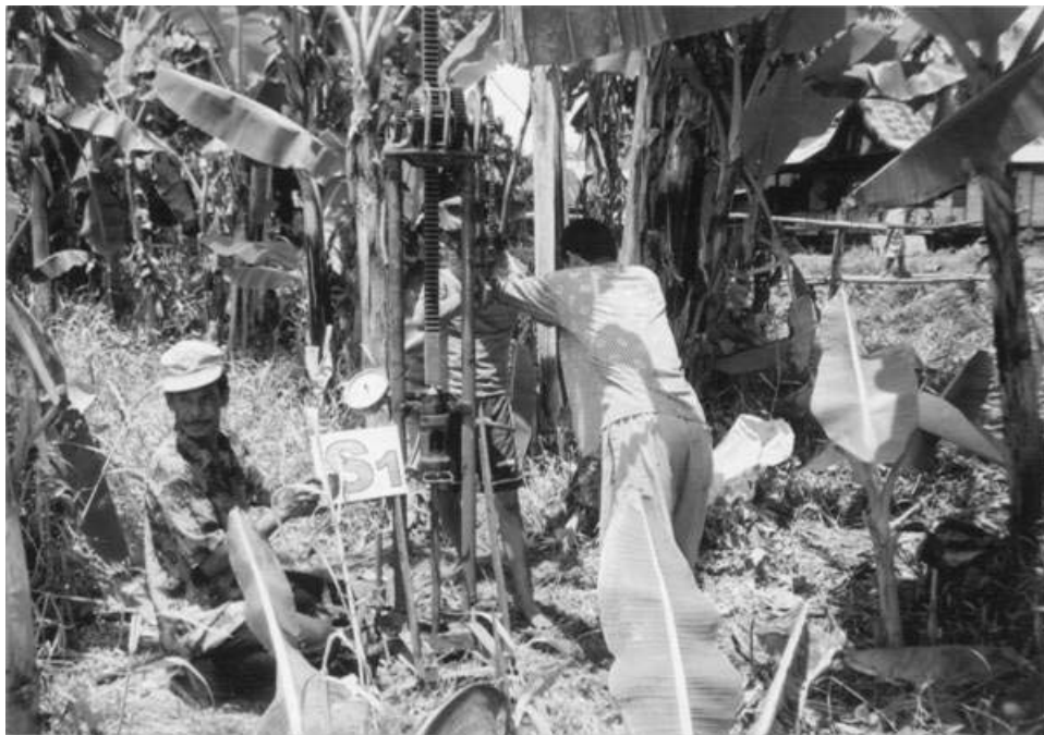
Gambar E-1.2 Uji Dutch Cone Penetration
