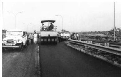
Asbuton Asphalt Construction at JabotabekCibinong, Bogor December 2003
