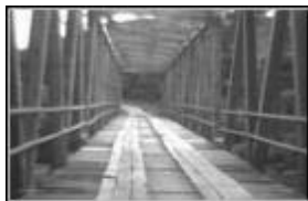
Bridge at Ondo-ondolu
