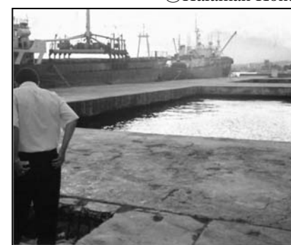
③ Drainase Rusak
