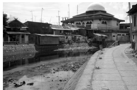
Polluted water in drainage canal
