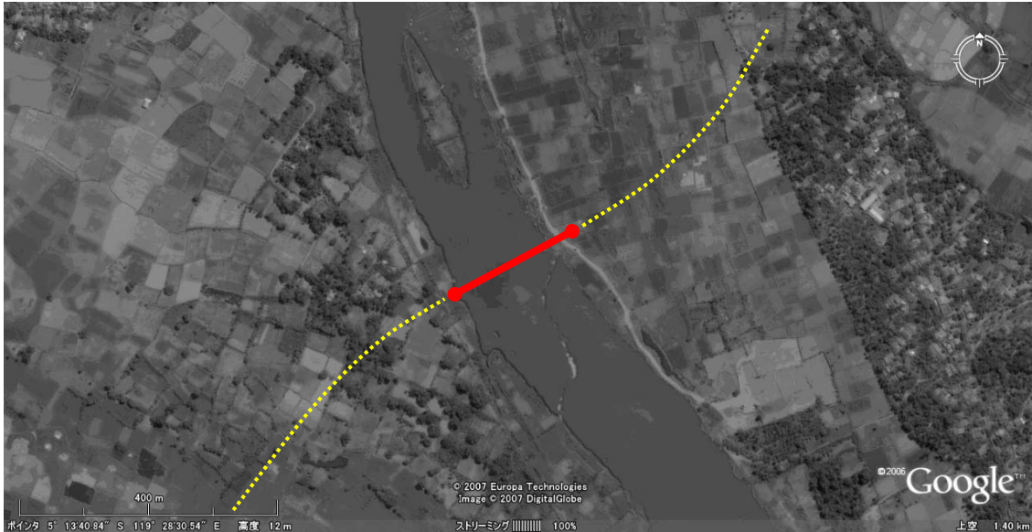
Figure F-3.5 Plane Photo of Jeneberang No.3 Bridge
