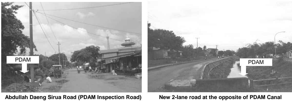
Figure 7.7.5 On-going Road Improvement for Section B
