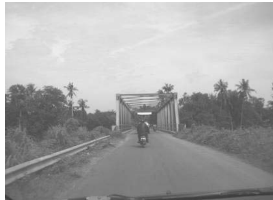
Bridge over Jeneberang River on Tj.Bunga -Takalar Road
