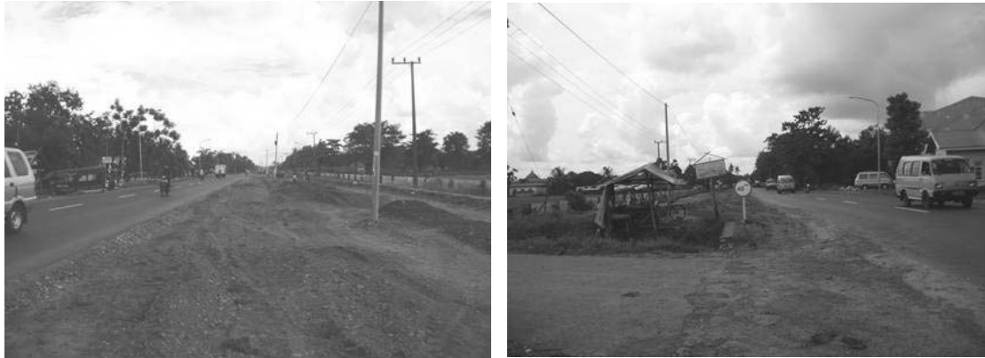
Figure 3.4.3 Trans-Sulawesi Road Widening Project by APBN (Maros-Pangkep)
