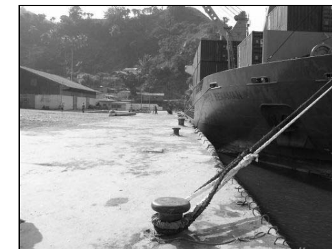
② Damaged berthing facility
