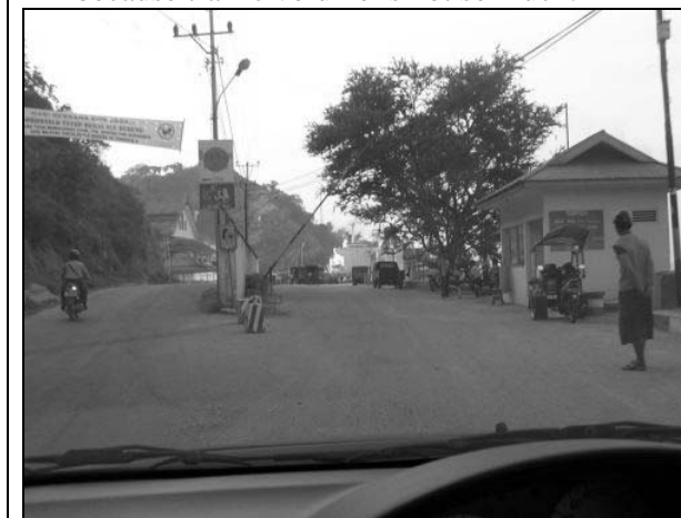
Road Condition around Gate of Port
