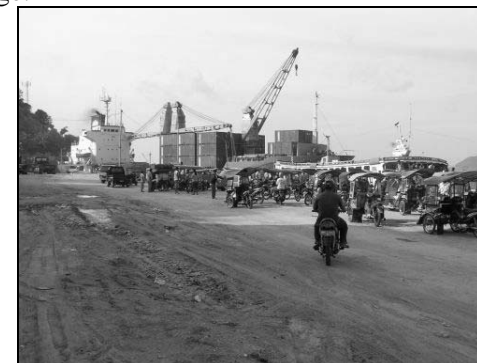
① Damaged pavement at access road and parking
