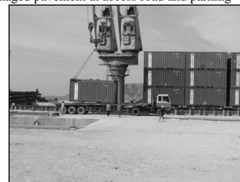
③ Unloading container by stevedoring crane
