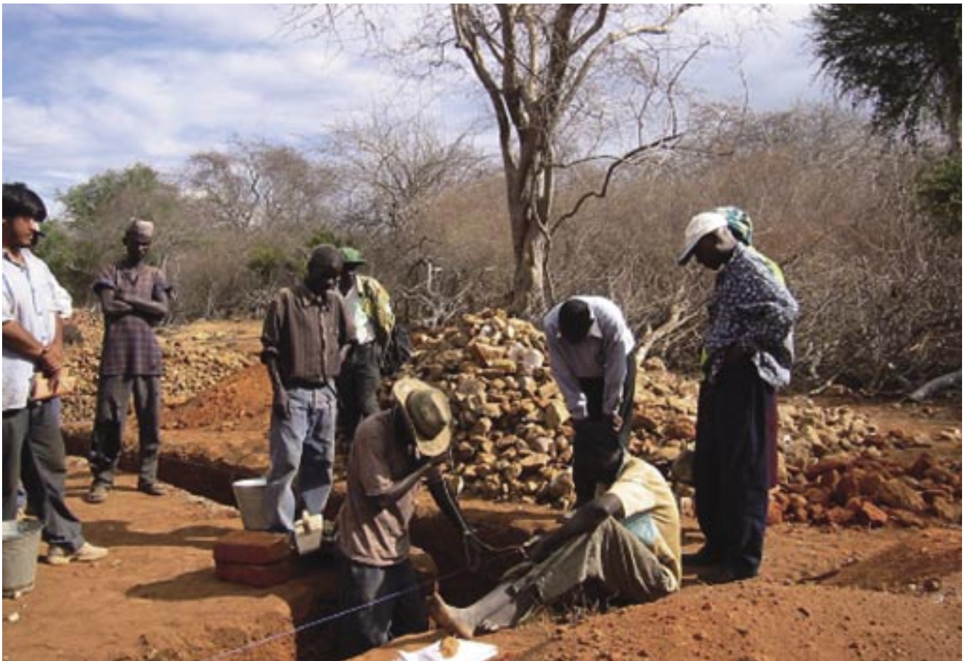
Parents working on the foundation of the classroom building.
