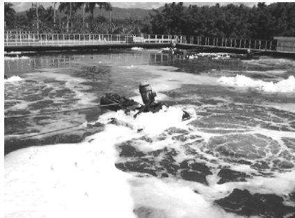
View of aerator in aeration pond in the Dominican Republic
