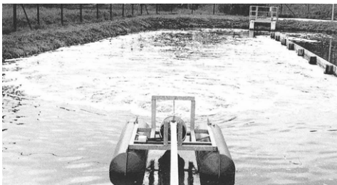
View of aerator in aeration pond in Indonesia
