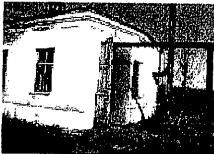
Building housing the chlorination equipment room Due to insufficient maintenance funds, deterioration of facility progresses
