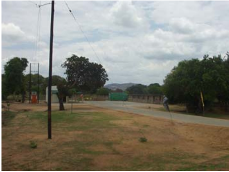
Overall view of the Michinoeki
