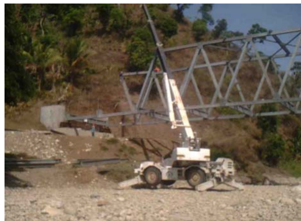
Usage of Crane of IGE at Actual Construction Site
