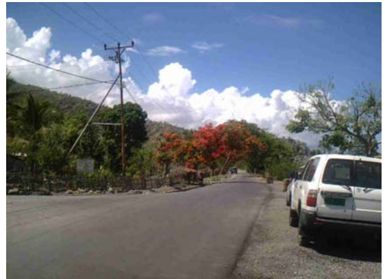
Road Condition after the Case Study
