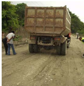
Proof Rolling Test for Sub-base Course
