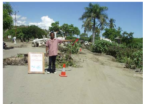
Safety for Traffic at Construction Site
