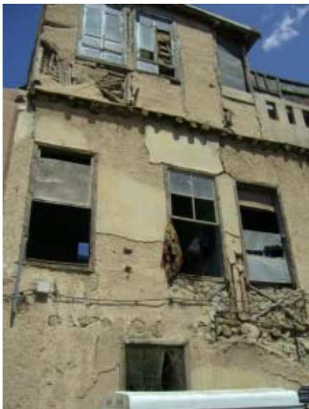
Straw is kneaded with cob and water added, and then dried in the sun and air. In the studio 1034, the surface of façade left for a long time without maintenance is ruined and consequently the units of clay and stone are exposed to rain, making the link mortar used between the units and stones crumble.
