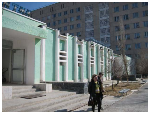
Entrance of administration office
