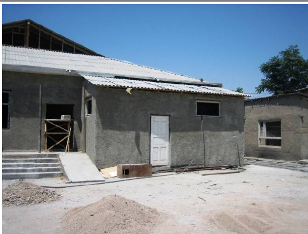
New Cancer Dispensary in Karmana Rayon, under construction
