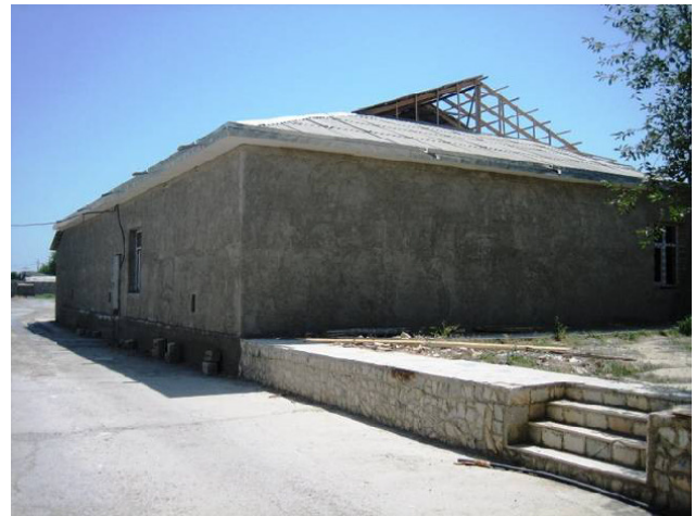
New Cancer Dispensary in Karmana Rayon, under construction
