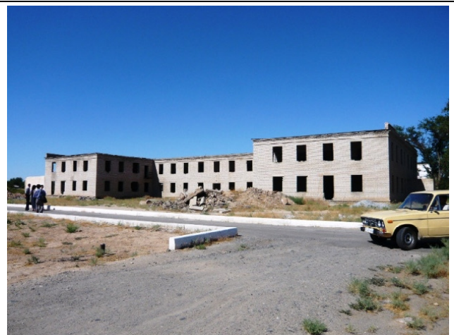
New building which is under constructed and will be established in 2008.
