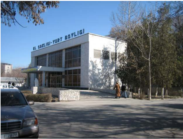
Entrance of main building
