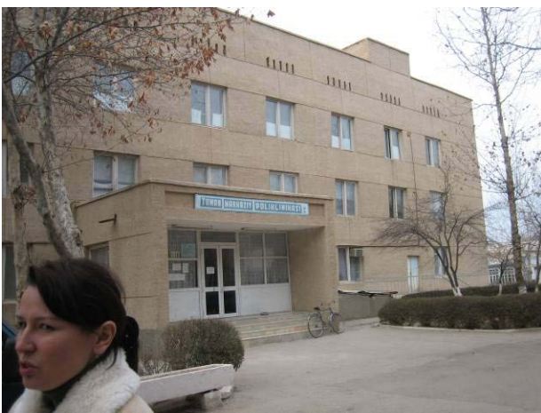
Inpatients Building, good maintained with flush toilet and sewage disposal
