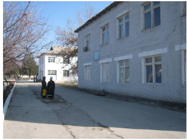
Surgical building (anterior) and Pediatrics building (posterior)
