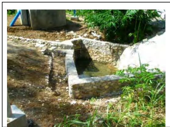
Spring Capture Site (After Construction)
