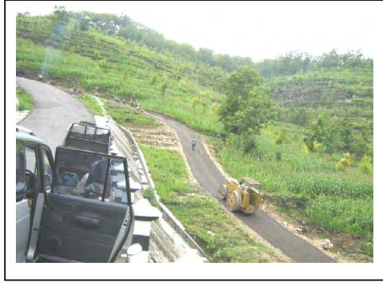
Access road (After Construction)
