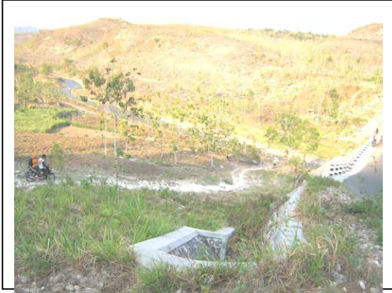
Access road (Before Construction)
