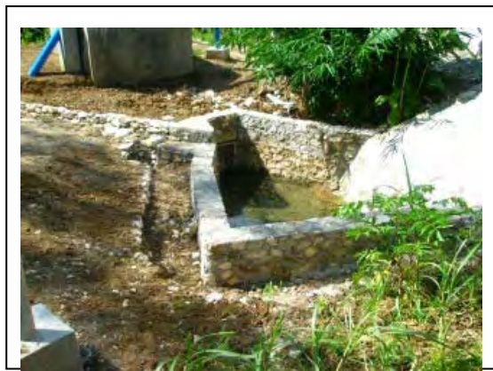
Spring Capture Site (After Construction)
