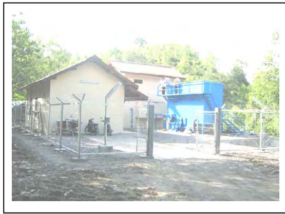
WTP Site (After Construction)
