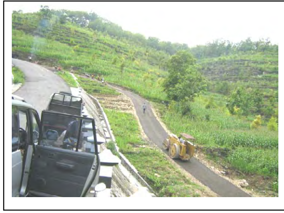
Access road (After Construction)
