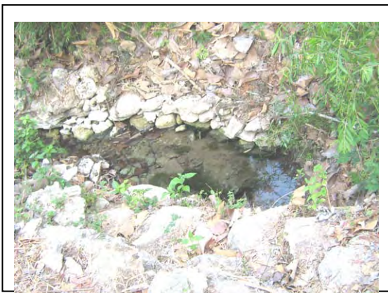
Spring Capture Site (Before Construction)
