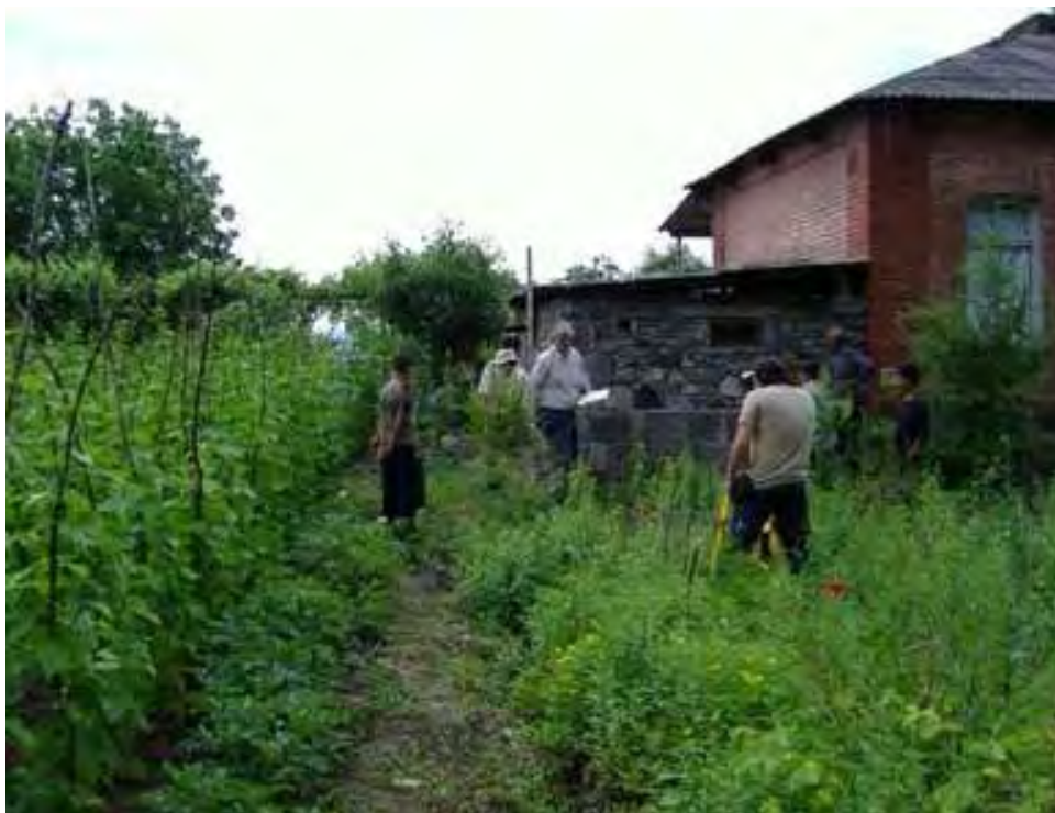
Figure 3.1.7 Leveling along the existing route
