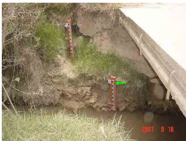
Photo S8-2-23 Setting level of electrode type water level gauge
