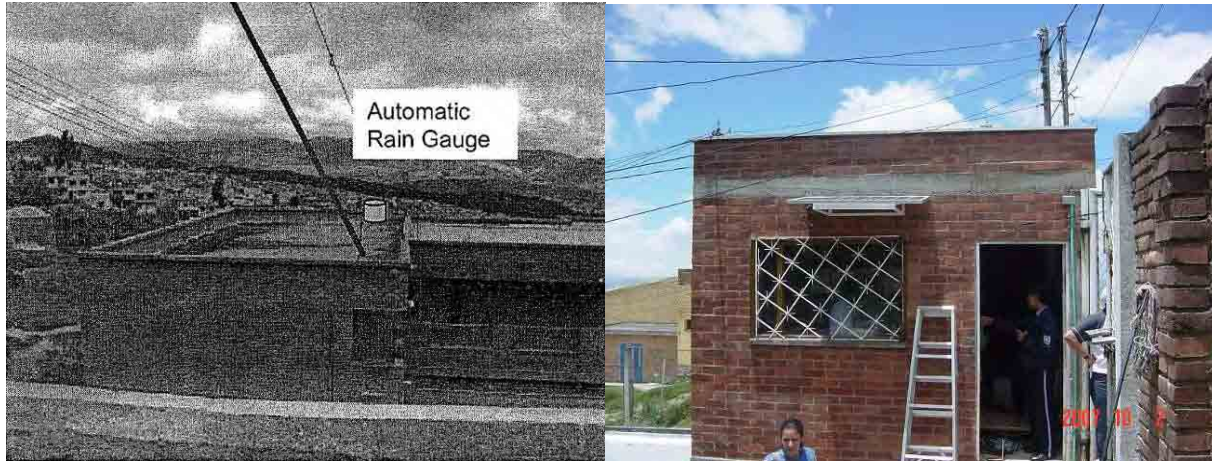
Photo S8-2-2 Rainfall gauge and Solar Panel in Moralba
