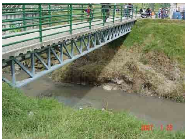
Photo S8-2-6 Footbridge for Ultrasonic Sensor installation
