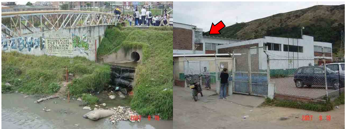
Photo S8-2-5 Staff Gauge (Left) and School's security guard house for Data Logger
