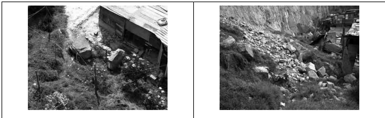
Photo S5-2-2 Rock Falls from Steep Slopes
