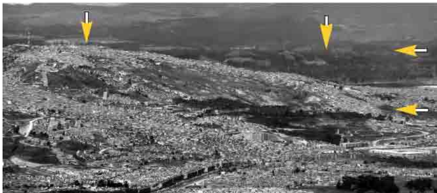
(a) from East Darker area at the center is the Landslide
