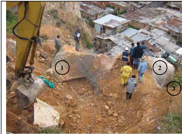
Termination of emergency measures for the block No.1
