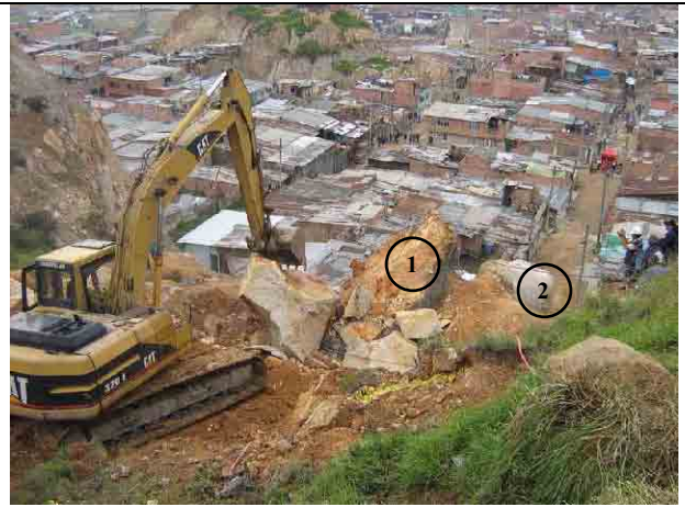
Remained pieces of block No.1 is removed with back-how
