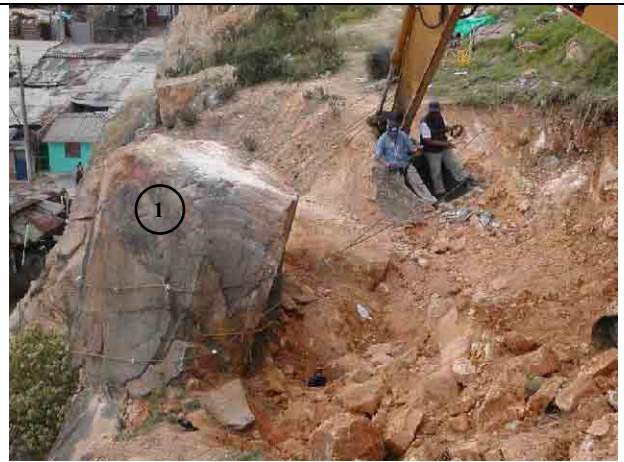
Wire net is fixed with wire rope
