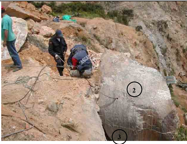
Installation of wire rope to blocks of No.2 and 3
