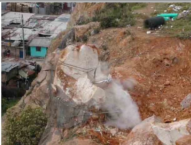
3rd blast of block No.1
