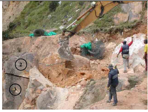
Removing of block No.2 after excavation of its back
