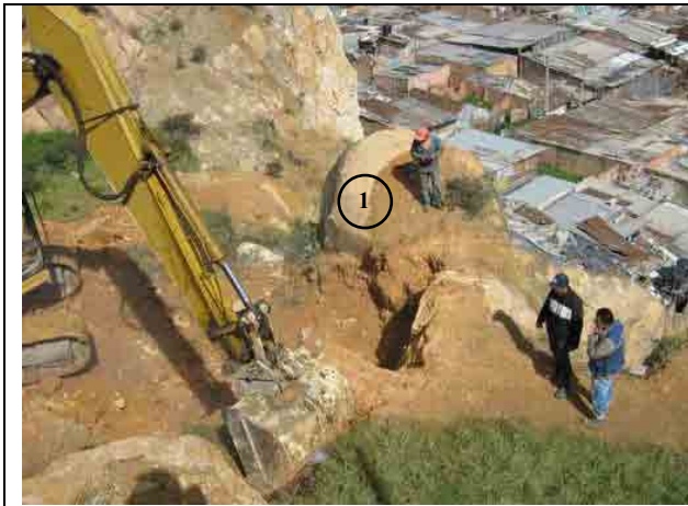
Excavation works behind the block No.1
