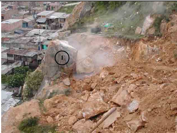
1st blast of block No.1 with white gun powder
