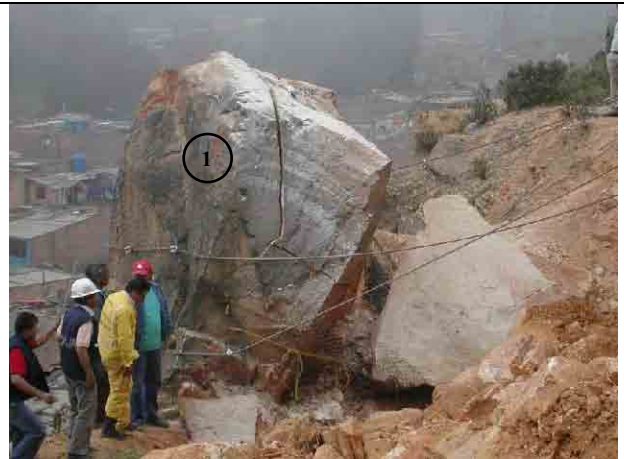
Wire net is fixed with wire rope
