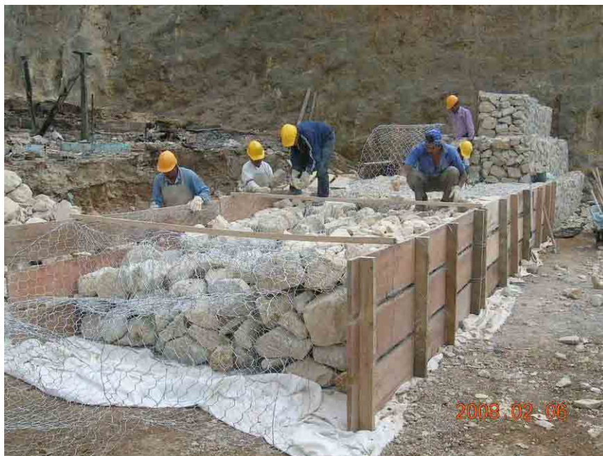
Photo 11-1 Local People Working Manually for Temporary Works
