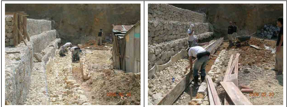
Figure 11- 20 Fixing of Cobble Stone by Concrete
