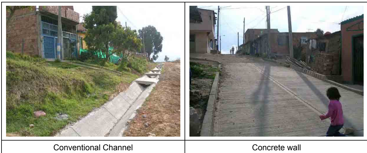
Figure 11- 22 Conventional Channel and Concrete Wall to be a Water Way Road in Rainy Season
