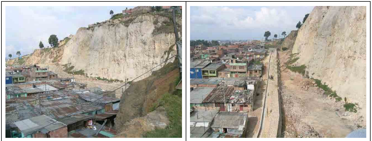
Figure 11- 17 General View of Temporary Works
