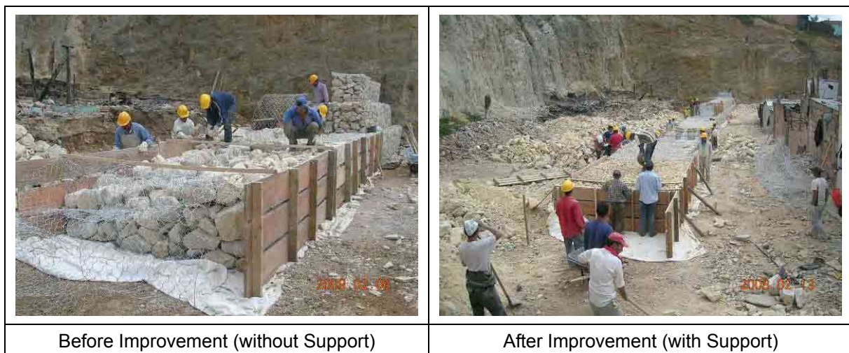
Figure 11- 25 Supporting of Form Work
