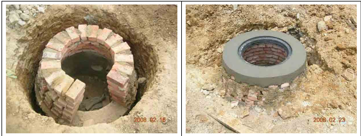
Figure 11- 21 Structure of Drainage Pit
