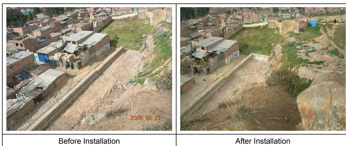
Figure 11- 19 Additional Protection Wall
