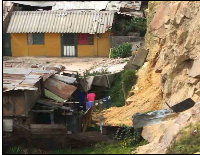
Photo 3-2 Homes Built in the Foothills Old Mine and Facing Landslide Hazards
