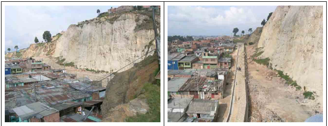
Figure 13-6 General View of Temporary Works
