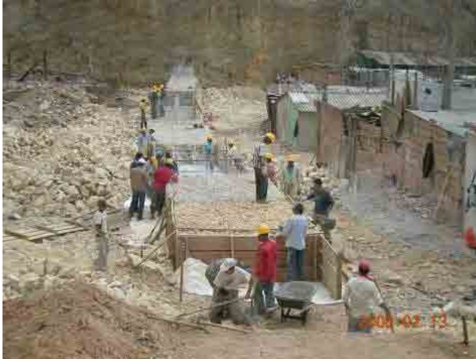
Photo 13-2 A lot of Local People working for the Temporary Works
