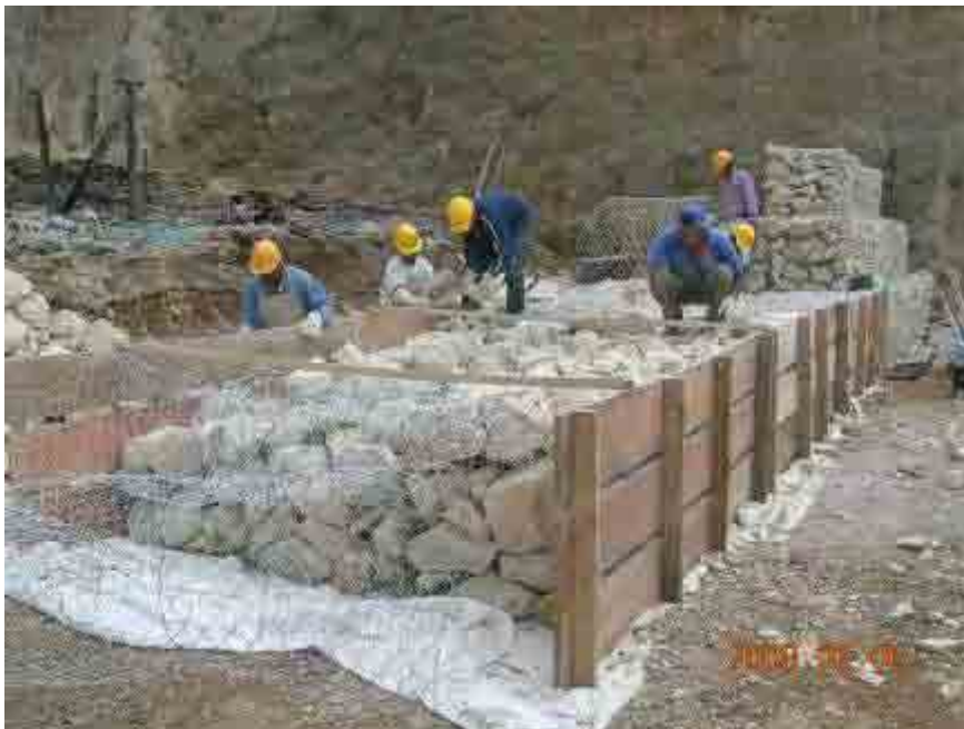
Photo 13-1 Local People working manually for the Temporary Works
