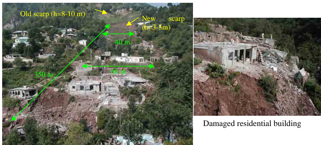
Figure 2.22 Recurrence of An Old Landslide (Landcreep) (Source: JICA Study Team)
