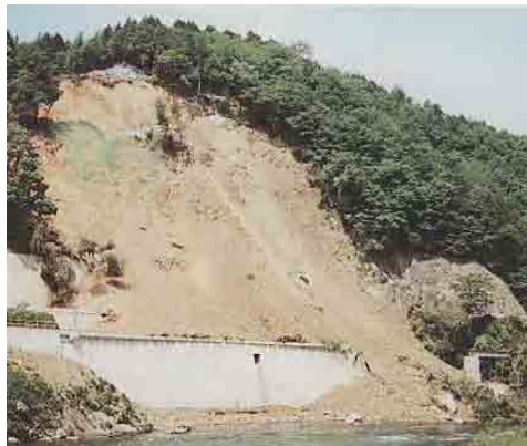
(a) After collapse
