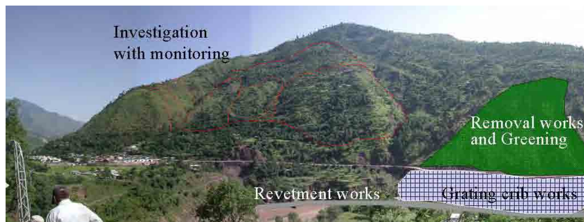
Figure 4.1.14 Counter measures against slope failures at the Naili area;
