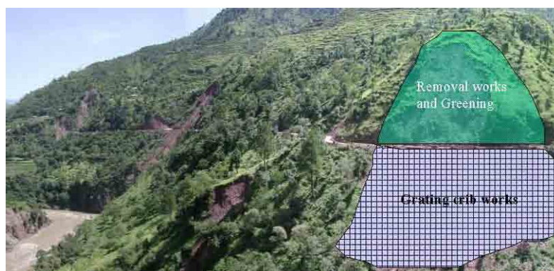
Figure 4.4.16 Recommendation on No.21 slope failure
