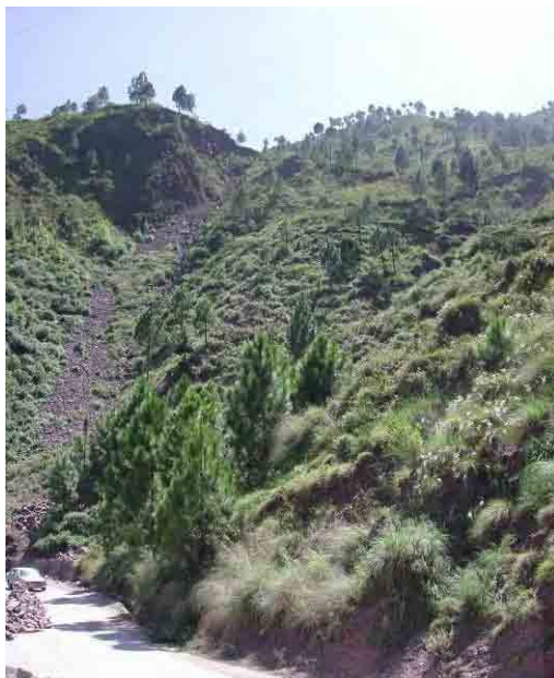
(C) Thick debris on a steep slope
