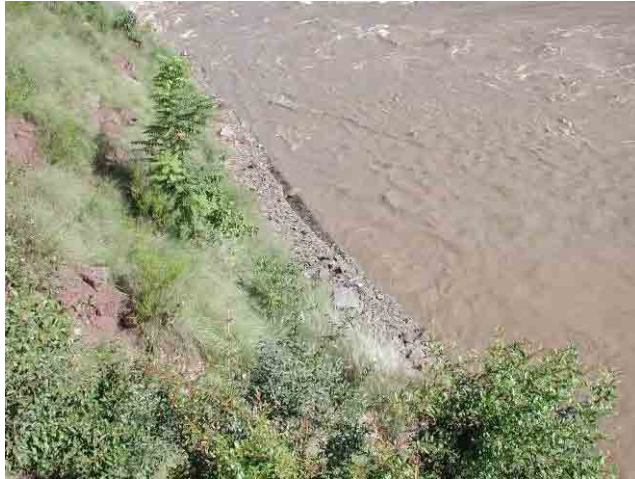
Photo 4.1.5 Gabion type revetment works near Supdgiran
