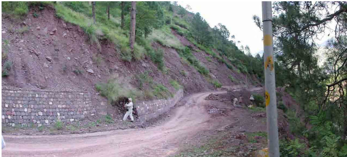
Photo 4.1.6 A Right flank of a landslide induced by a road construction near Jaskool
