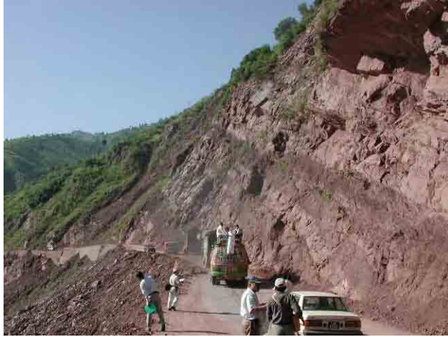
(B) Crack rich sandstone
