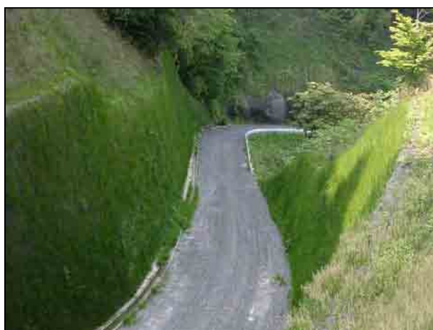
Photo 4.1.7 Greening works on steep rock slope
