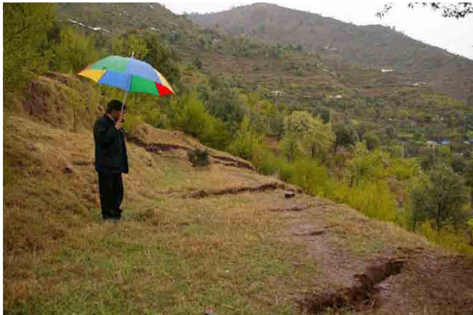
Photo.3.5.3 Tension cracks developed on the flexural scarp
