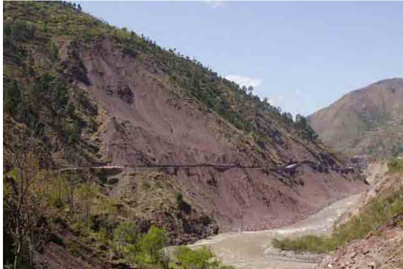
Photo.3.5.11 Active landslide due to under cutting and civil works at Jaskool
