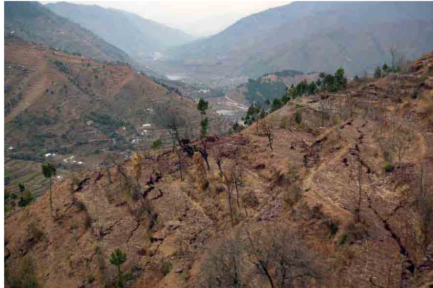
Photo 3.2.1 A series of tension cracks developed on a slope parallel to the active fault
