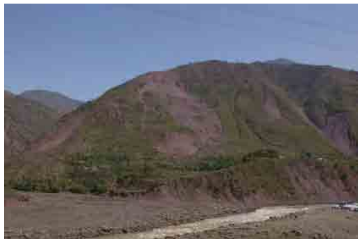
Photo 3.5.2 Slope failures (shallow landslide) at Kulori
