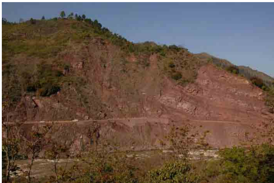
Photo.3.5.7 Large slope failure on under cut slope at Sugli
