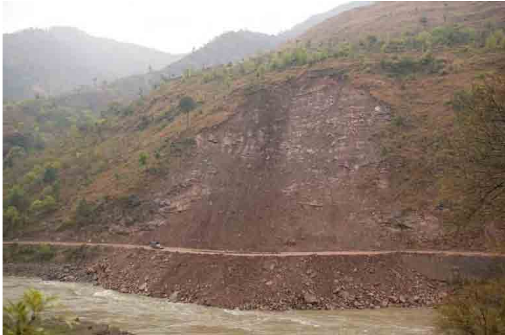
Photo 3.5.9 landslide on anti-dip slope at Badihara
