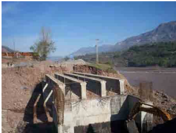
PC girders erected
