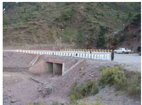
No.5 Bridge site, completed
