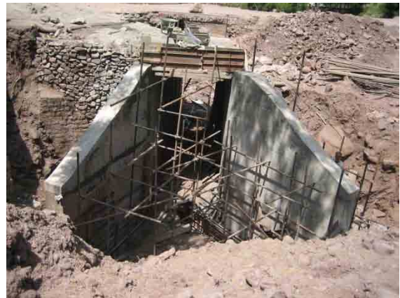
Wing wall under construction
