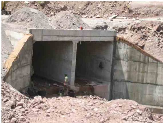
Wing wall under construction
