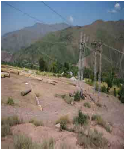
Top of the slope before cutting
