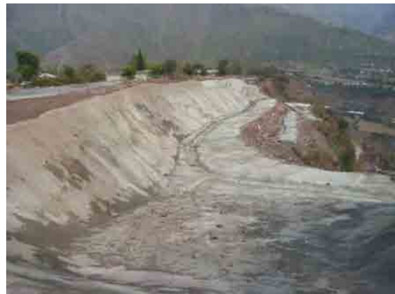
Mortar spray and Concrete cover work
