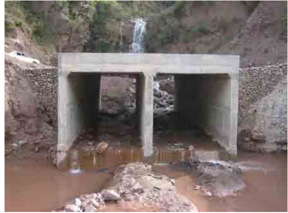
Box-culvert, completed
