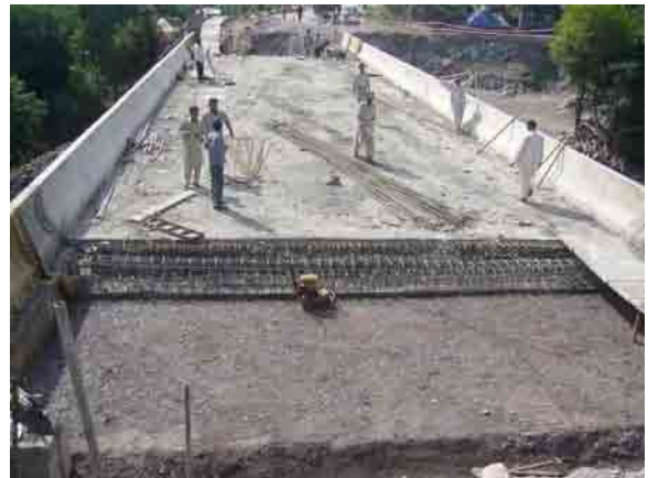
Super structure constructed
