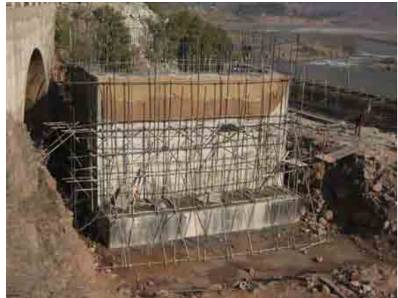
An abutment under construction
