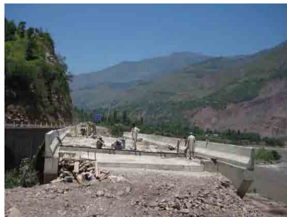
Super structure constructed
