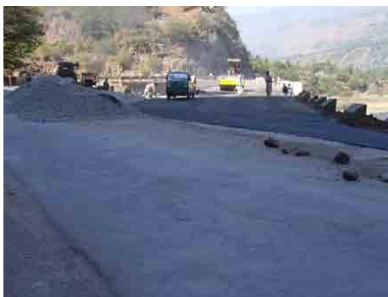
Asphalt pavement on the bridge
