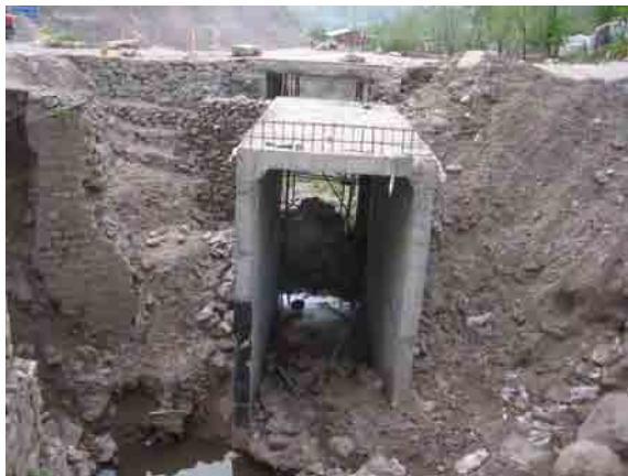
Box-culvert, completed
