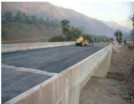
Asphalt pavement on the bridge
