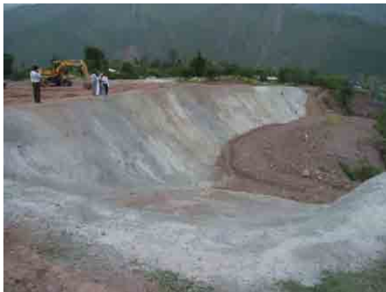
Slope protection (Mortar spray), completed
