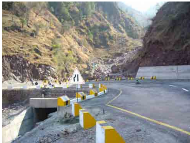
No.3 Bridge site, completed
