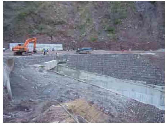
Road works, embankment protected by gabions
