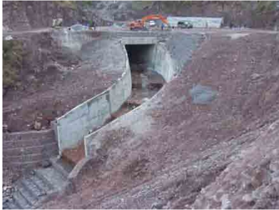
Log chute, under construction
