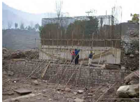
An abutment under construction
