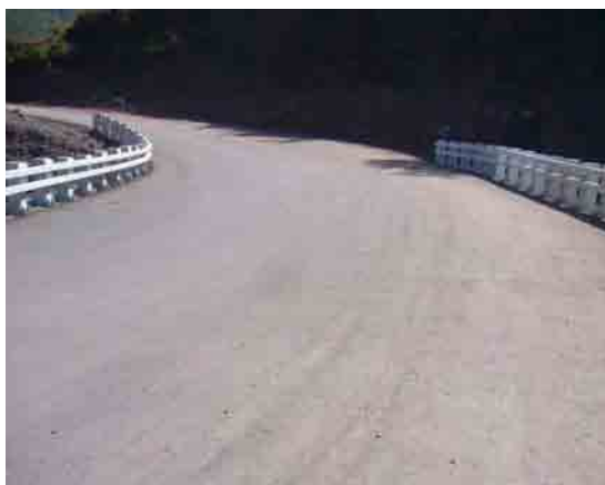
Asphalt pavement, completed
