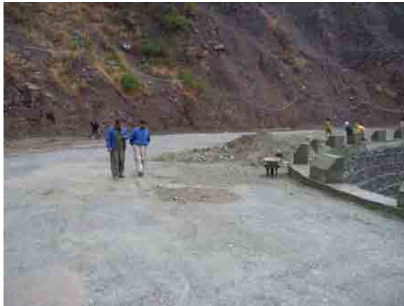
Base cause laying
