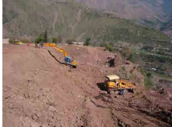
Sloping work under cutting
