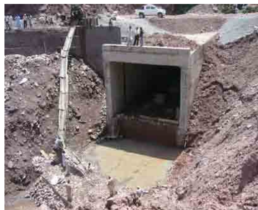
Box-culvert, completed
