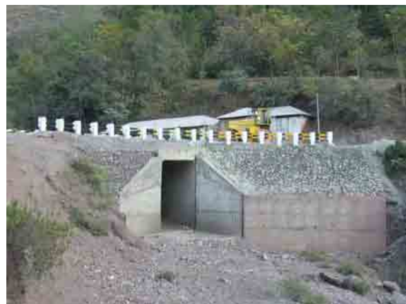
No.4 Bridge site, completed
