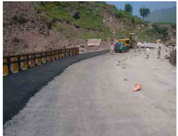
Asphalt pavement work
