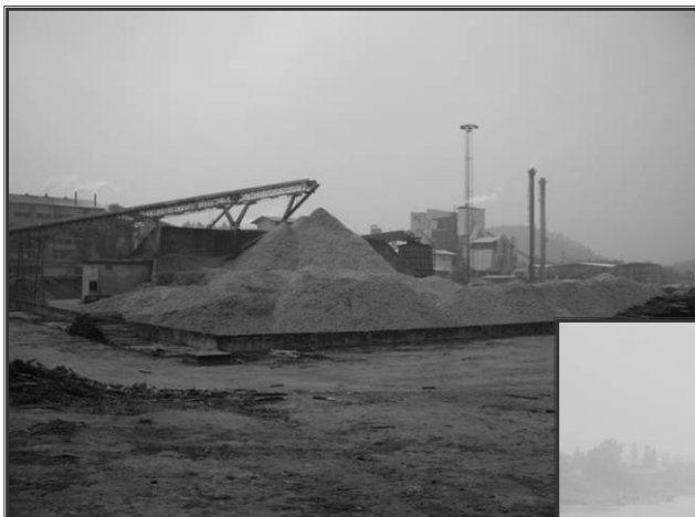
Photo No. 3.1 Wood chip factory at paper mill
