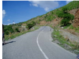
Photo: Arterial road (A01) under improvement
