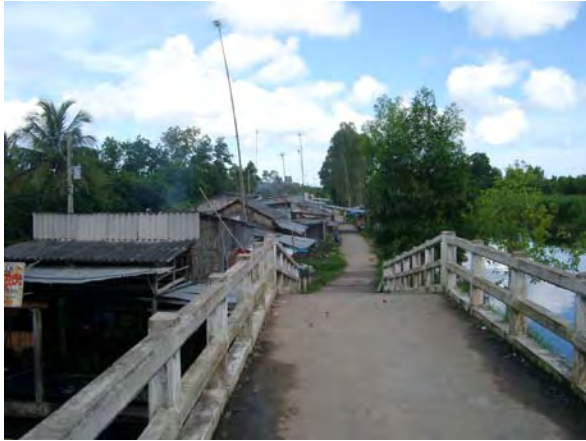
R-14b: Subject site for widening of the existing road
