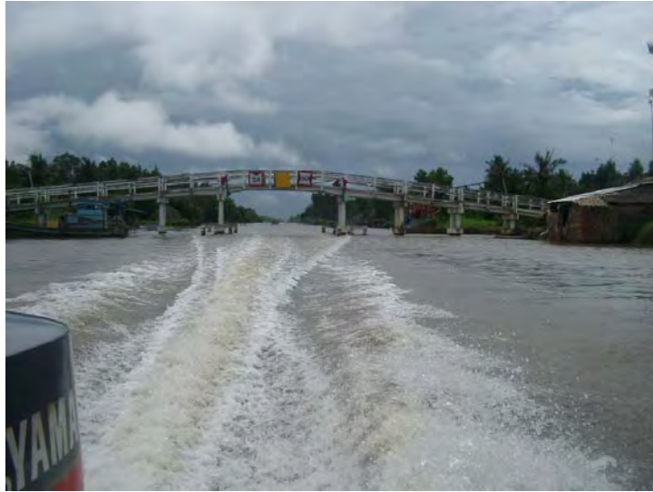
A bridge over a relatively wide canal: 2.8 m clearance between the girder and the water level is secured to allow navigation.
