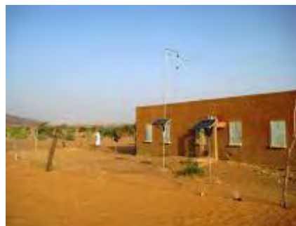
Fence for the protection of the radio system (N'Titam)
