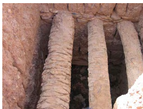
It is easy to flow out the excrement by rain water and to weather.
