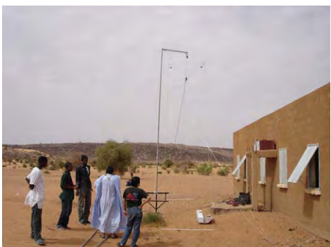
Installation of the radio transmission (health center)
