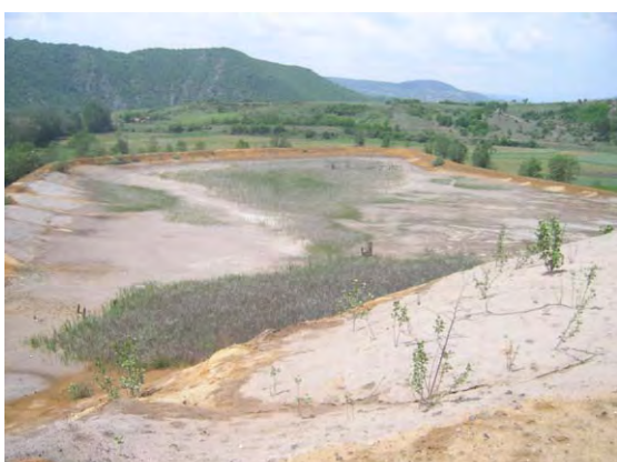
View of the old tailing dam on the Cu side of Suva Ruda Mine
