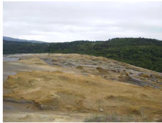
Erosion of Tailings Dam
