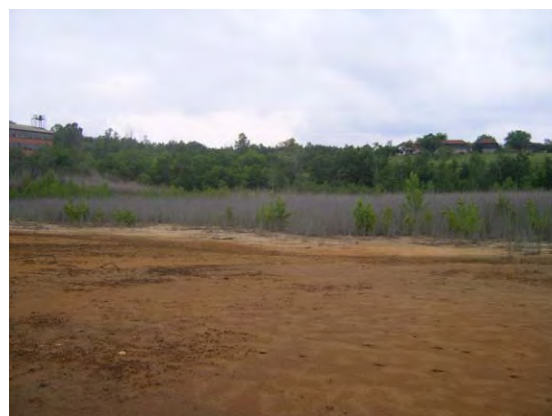
Tailing dam No. 3 at Lece mine
