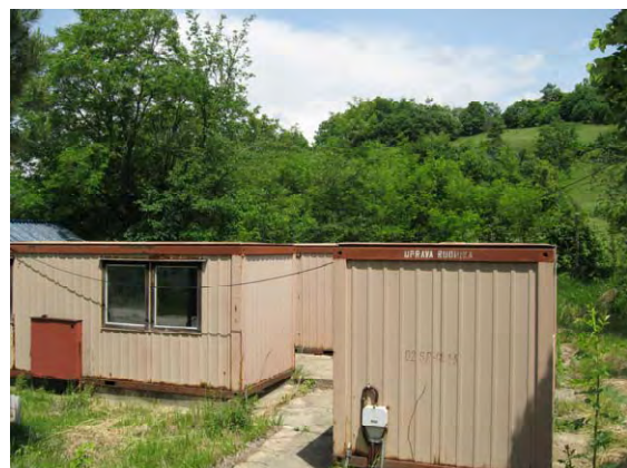
A mine office and locker-rooms near the maintenance shop.
