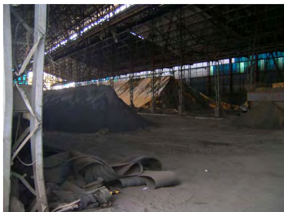
Concentrate storage house
