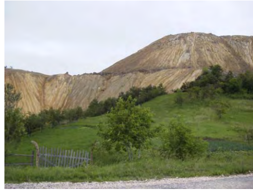
Erosion of Waste Dump
