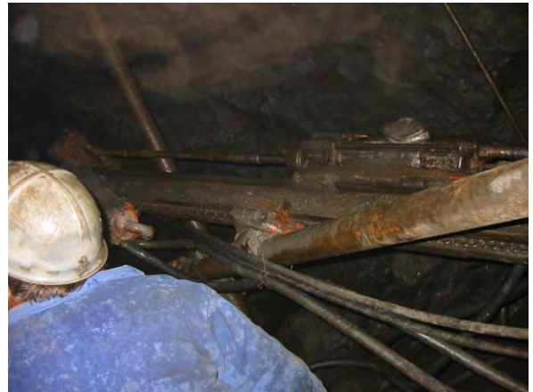
A drill machine in operation at an underground stope. It is dark and dirty.
