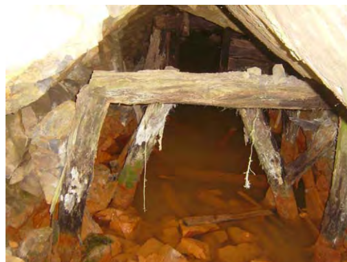
Prospecting adit in intermediate zone of the Kizevak deposit
