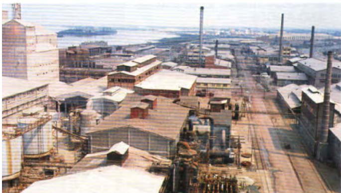
Exterior of the smelting plant
