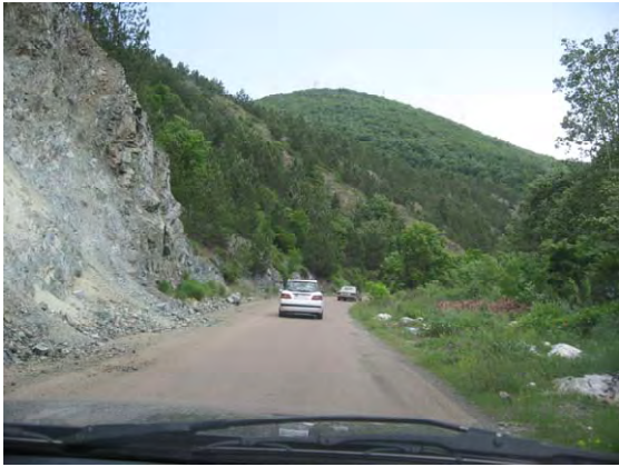
A 6km paved access road to the pit from the national road. This road was constructed by the mine in 1984.
