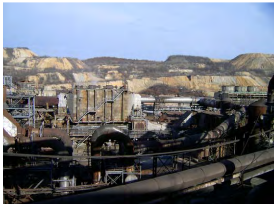
Smelter over view
