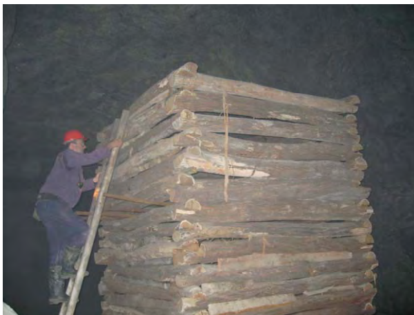
Tailings materials from the processing plant are used to fill the mined space for cut & fill method stopes. Water in tailings is discharged by this chimney.
