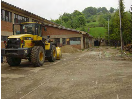
An entrance of the Grot Mine (1,300m level)
