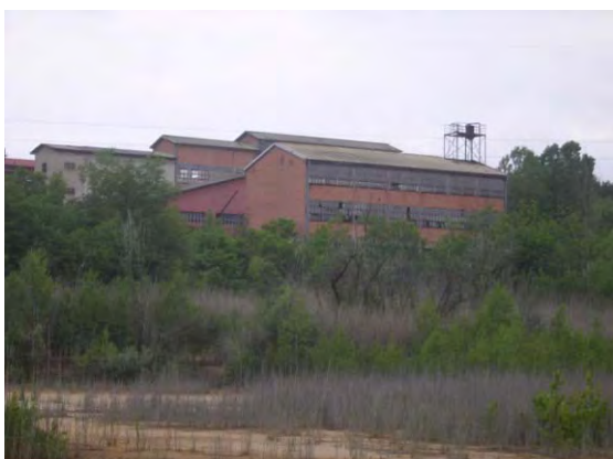
Mineral processing plant at Lece mine
