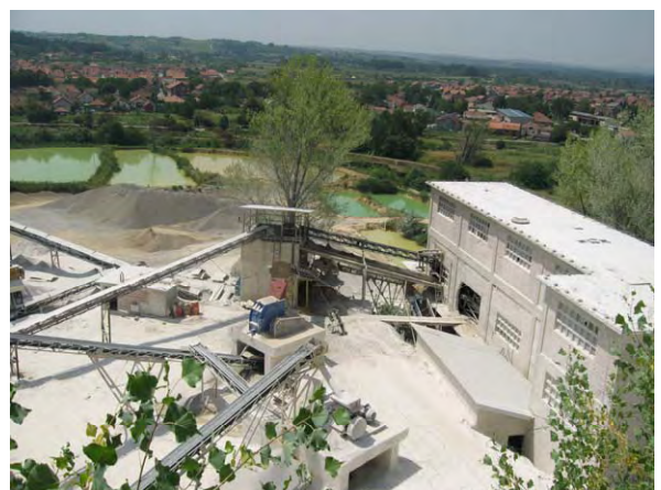
The crushing plant can produce various sized products. there are sedimentation ponds to clarify dirty water.
