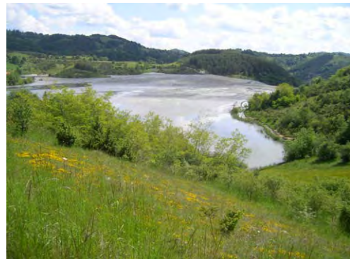
View of Tailing dam at Grot mine
