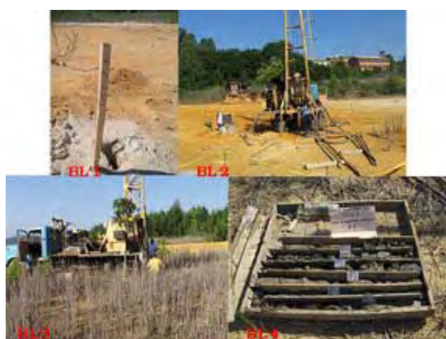
Fig.7.16 Core Drilling Points at the Lece Mine Tailings Dam
