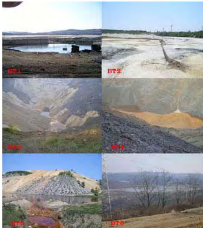
BT-1 : Oldest tailing dam of RTB-Bor, • BT-2 : Old tailing dam for Case Study (CS: core-drilling and sampling) • BT-3, BT-4 : Permeable water in the open pit, • BT-5 : Acid seepage from Over Burden stock yard (strong acid of pH2.6), • BT-6 : Operating tailing dam No.1 (front), No.2 (behind)
