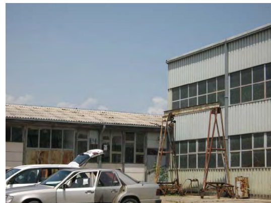
Repair shop (R) and warehouse for spare parts (L)
