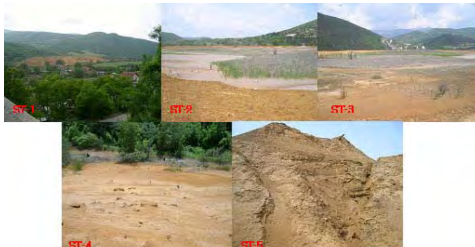
• ST-1 : Suva Luda mine tailing dam (Right : Pb-Zn flotation tailing dam, Left : Cu flotation tailing dam) • ST-2 : Pb-Zn flotation tailing dam, • ST-3 : Cu flotation tailing dam, ST-4 : Underground water monitoring holes on the bank, • ST-5 : Erosion trace on the bank
