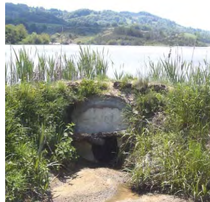
Collector Pipe of the Tailings Dam
