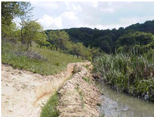
Street gutter around the Tailings Dam
