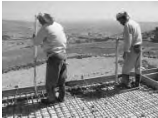
Concrete Compacting for Wall of Ground Water Tank (50m 3 )
