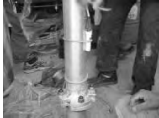
Installation of Electric Wire and Water Level Probe
