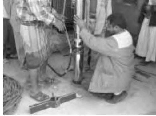
Installation of Submersible Motor Pump
