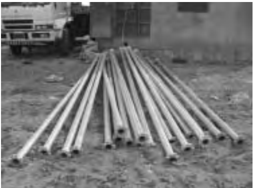
Column Pipe to be installed
