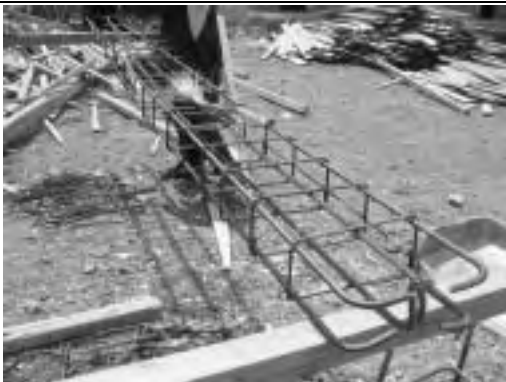
Rebar Bending at Stock Yard
