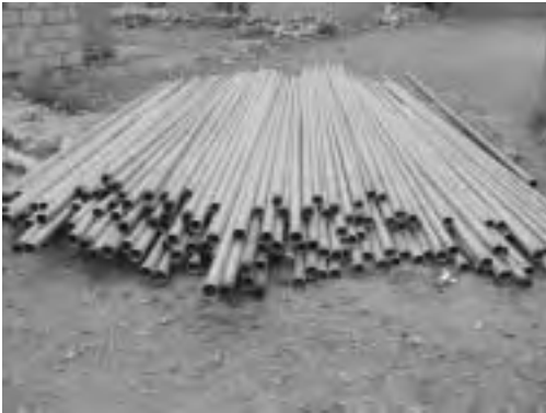
Pipeline in Stock Yard
