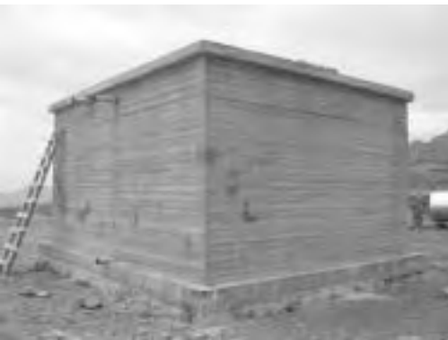
Ground Water Tank (50m 3 ) after Concrete Work
