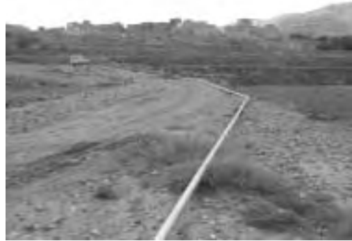
Installed Pumping Main (3")
