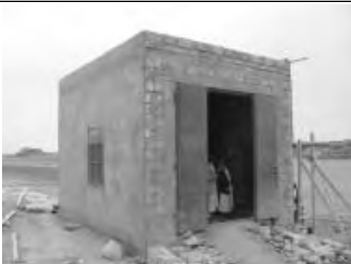
Existing Pump House under Rehabilitation
