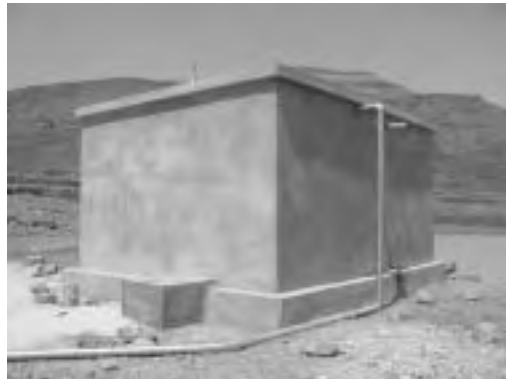
Ground Water Tank (50m 3 ) after Plastering Work
