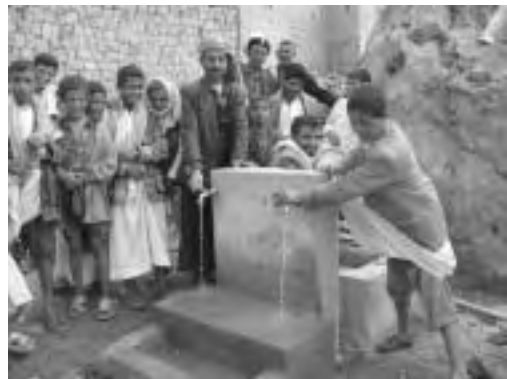
Constructed Public Fountain
