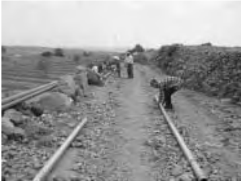
Installation of Pumping Main (3")
