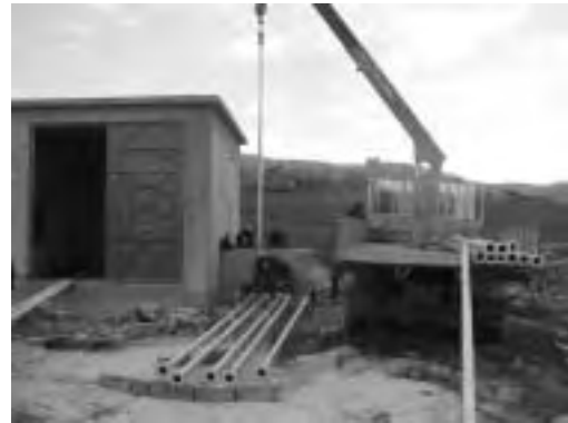
Installation of Column Pipe
