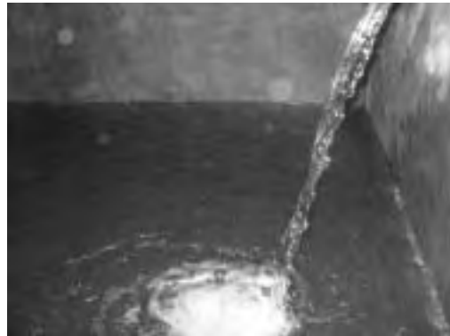
Water Flowing in Constructed Ground Water Tank (50m 3 )
