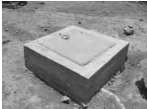
Valve Chamber along Distribution Main
