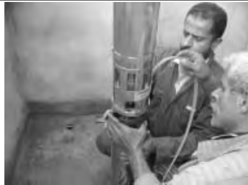
Installation of Submersible Motor Pump
