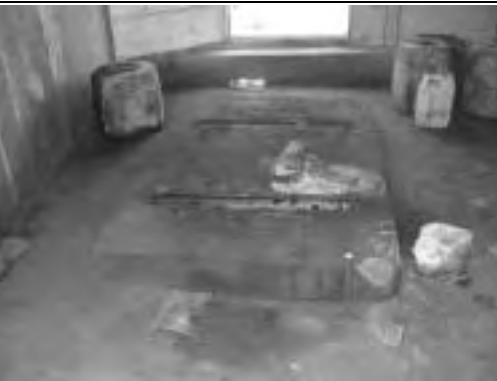
Foundation after Removal of Diesel Engine for Well
