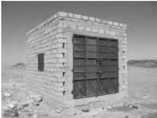
Existing Pump House constructed by Community
