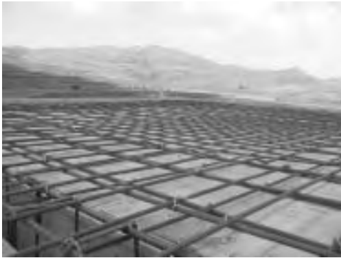
Reinforcing Rebar for Beam and Roof of Pump House
