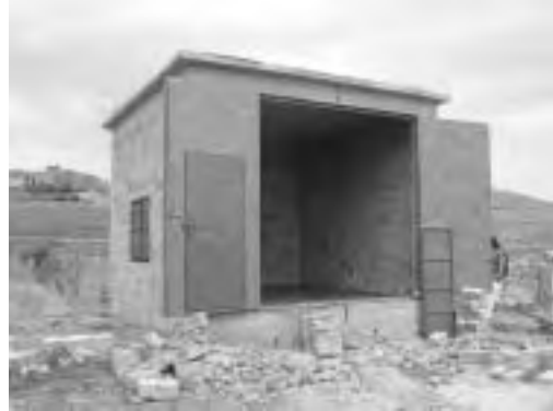
Door and Windows for Pump House
