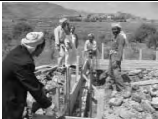
Reinforced Concrete Work for Underground Beam of Pump House
