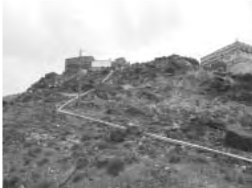
Installed Pumping and Distribution Main to/from Water Tank
