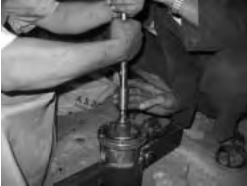
Installation of New Column Pipe for Well
