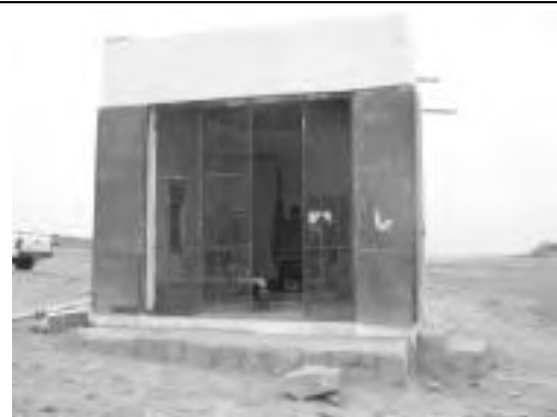
Rehabilitated Existing Pump House
