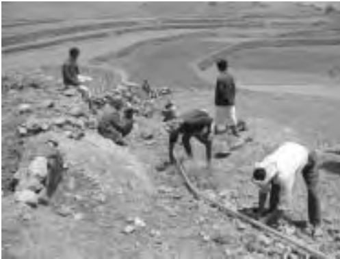
Installation of Distribution Main (1.5")
