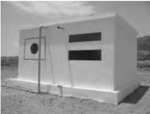
Constructed Ground Water Tank (50m 3 )
