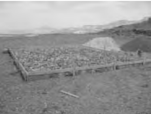
Crushed Stone for Foundation of Ground Water Tank (50m 3 )
