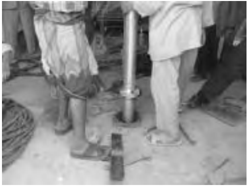
Installation of Column Pipe
