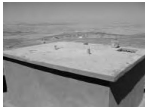
Rooftop of Existing Ground Water Tank (25m 3 )
