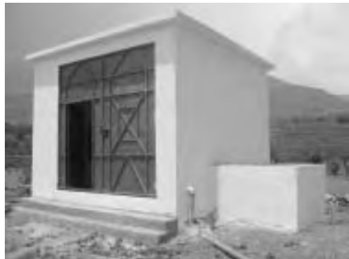
Constructed Pump House and Pit
