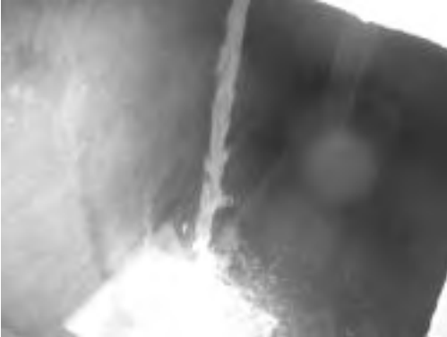
Water Flowing in Existing Ground Water Tank
