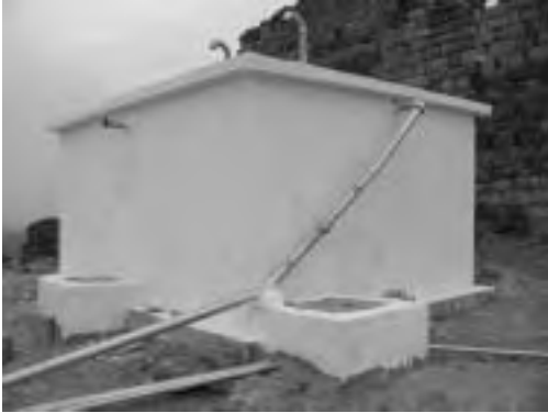
Rehabilitated Existing Ground Water Tank (25m 3 )
