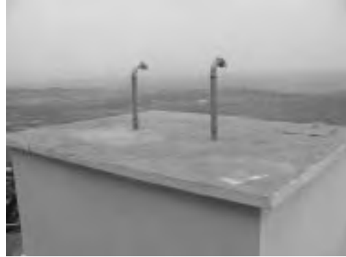
Rehabilitated Rooftop of Existing Ground Water Tank (25m 3 )
