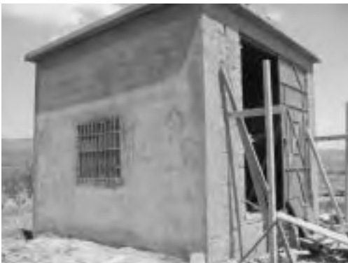
Plastering Work for Pump House
