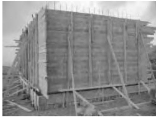
Formwork for Wall of Ground Water Tank (50m 3 )
