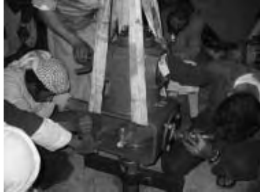
Installation of New Drive Unit for Well
