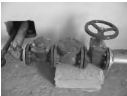
Accessories (from left: Pressure Gauge, Water Meter, Check Valve and Gate Valve)
