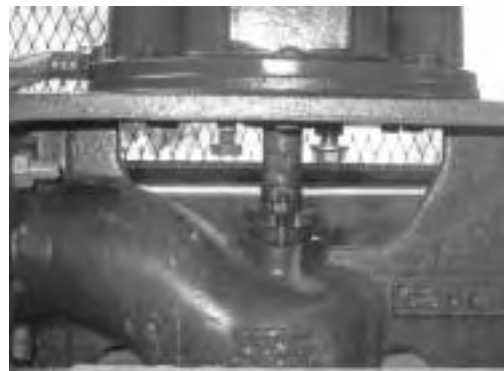
Gland Nuts of Pump for Well
