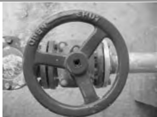
Gate Valve Adjustment (Clockwise - Shut, Anti-clockwise - Open)
