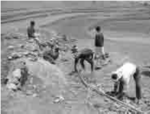
Installation of Distribution Main (1.5")
