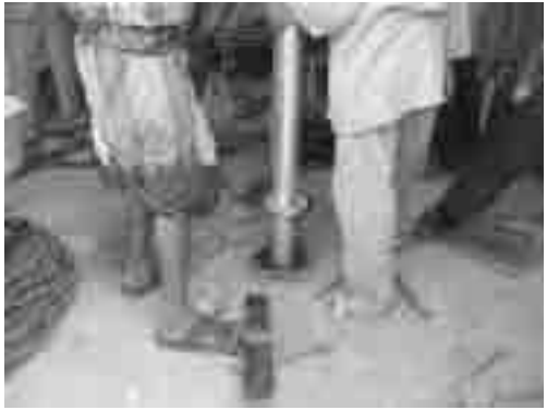
Installation of Column Pipe
