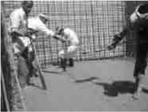
Concrete Casting for Floor of Ground Water Tank (50m 3 )
