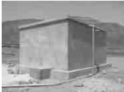
Ground Water Tank (50m 3 ) after Plastering Work
