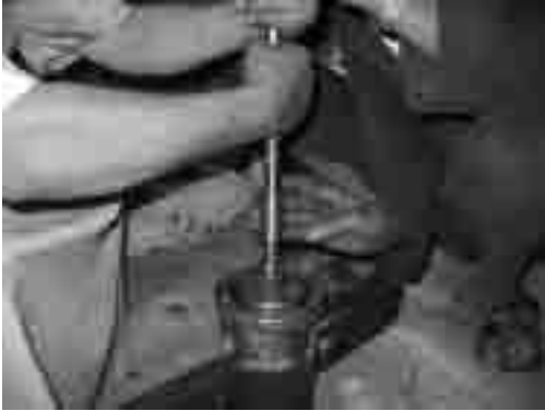
Installation of New Column Pipe for Well
