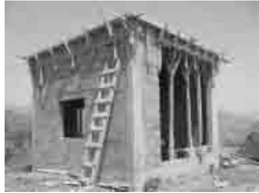
Reinforced Concrete Work for Beam and Roof of Pump House
