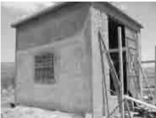
Plastering Work for Pump House
