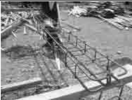
Rebar Bending at Stock Yard
