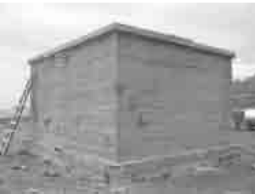
Ground Water Tank (50m 3 ) after Concrete Work
