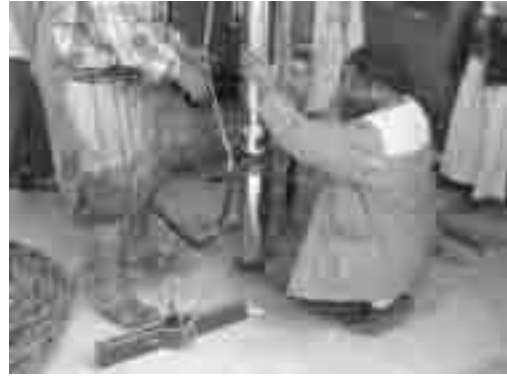
Installation of Submersible Motor Pump
