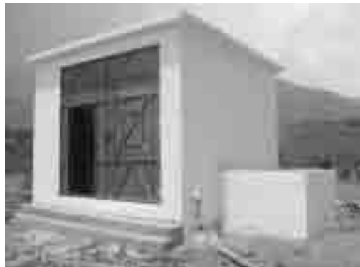
Constructed Pump House and Pit
