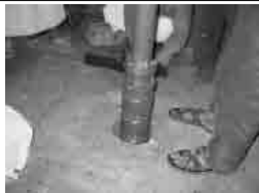
Installation of New Vertical Shaft Pump for Well
