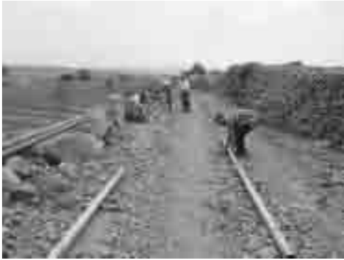
Installation of Pumping Main (3")
