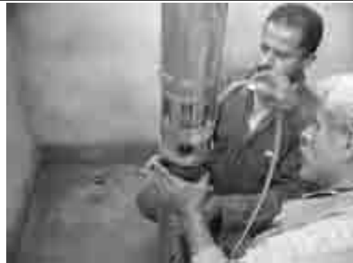
Installation of Submersible Motor Pump
