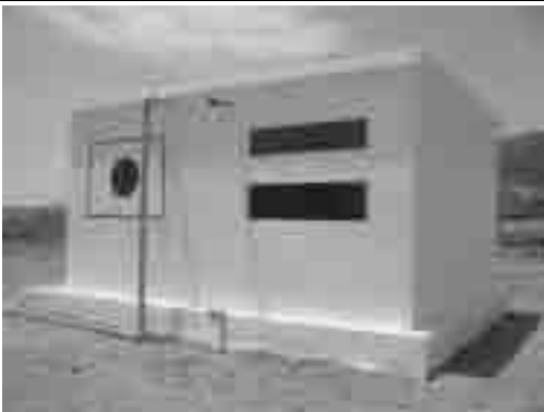
Constructed Ground Water Tank (50m 3 )
