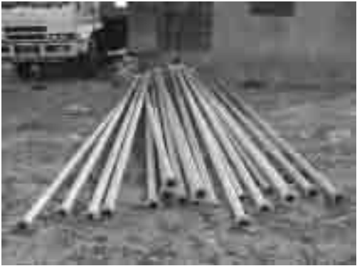
Column Pipe to be installed
