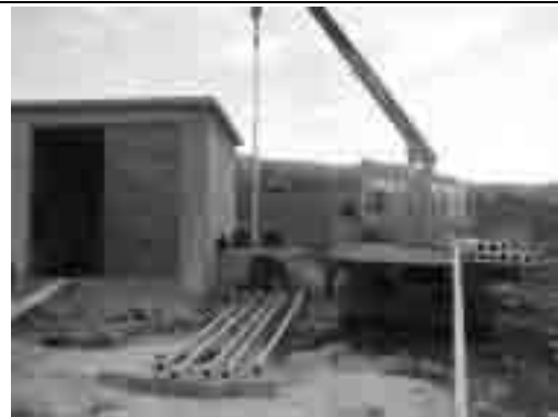
Installation of Column Pipe
