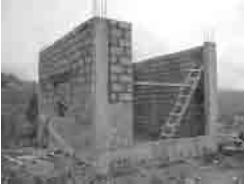
Masonry Work by Concrete Block for Wall of Pump House
