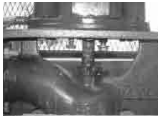
Gland Nuts of Pump for Well
