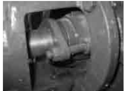
Gland Nuts of Pump for Booster
