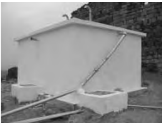
Rehabilitated Ground Water Tank (25m 3 )
