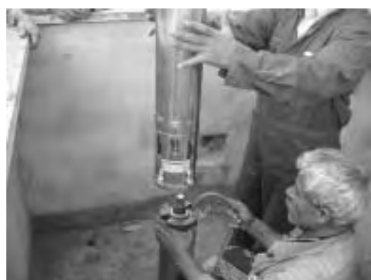
Installation of Submersible Motor Pump
