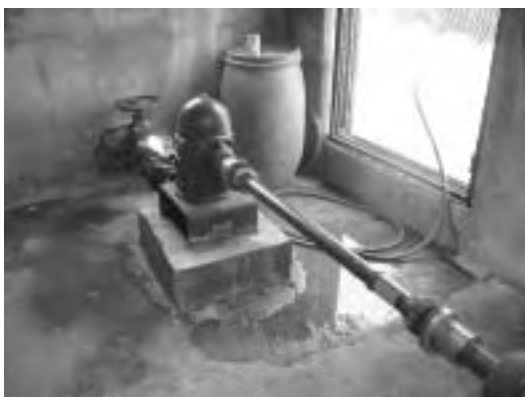
Well Pump after Replacement
