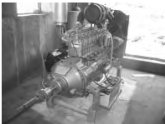
Replaced Diesel Engine for Well Pump
