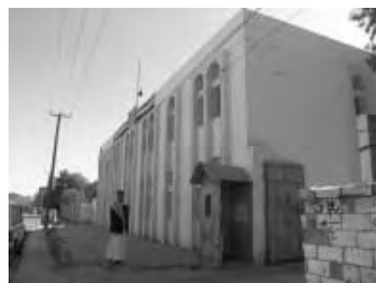
GARWSP Sana'a Branch Office
