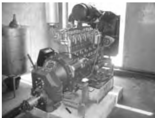
Replaced Diesel Engine for Booster Pump
