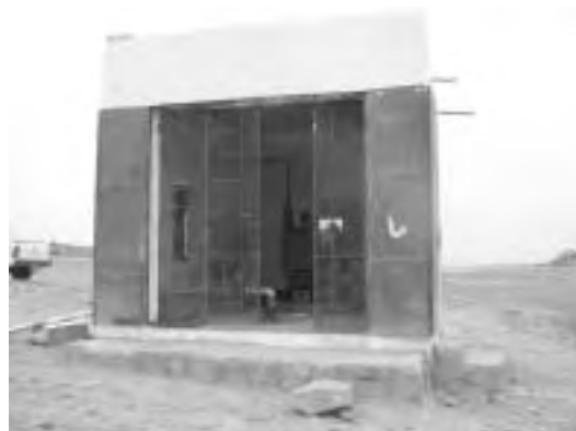
Rehabilitated Pump House
