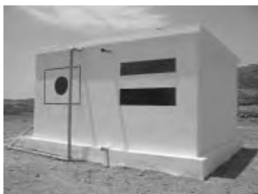
Constructed Water Storage Tank (50m 3 )
