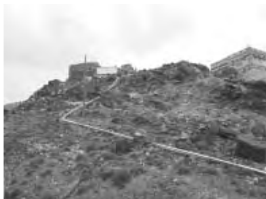
Installed Pipeline (Pumping & Distribution Main)
