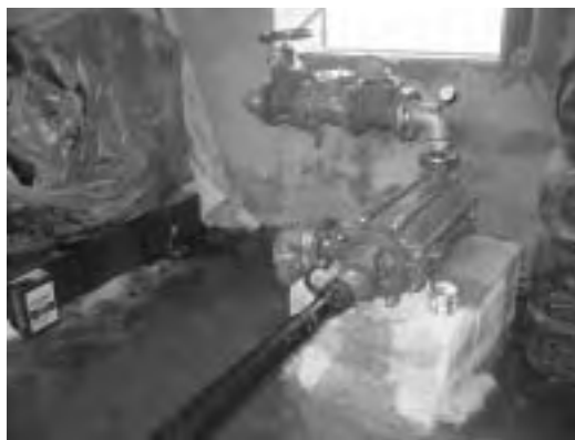
Booster Pump after Replacement
