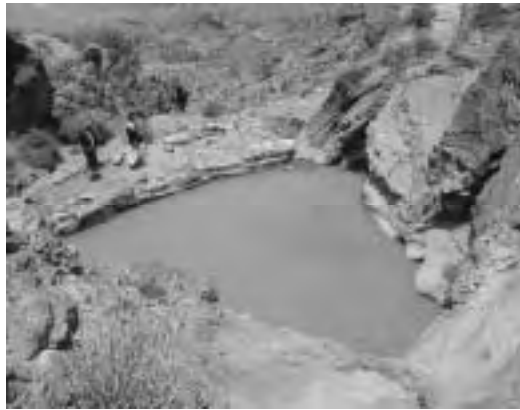
Cistern for Collecting Rainwater
