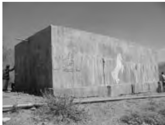
Existing Water Storage Tank
