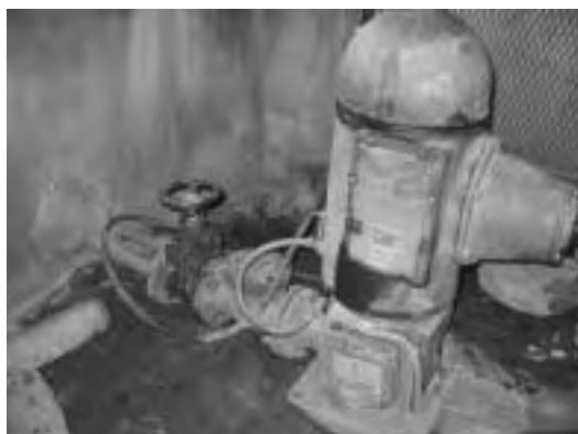
Well Pump before Replacement
