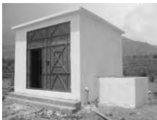
Constructed Pump House with Pump Pit
