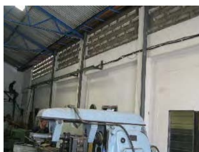
Installation of a new cable rack
