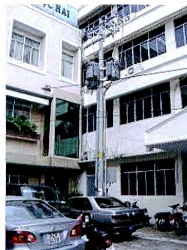
Figure 3. Completion of the low voltage post
