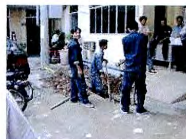
Figure 2. Installation of the power line
