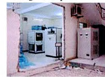
F.9 Installation of equipment 3
