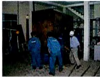
F.8 Installation of equipment 2
