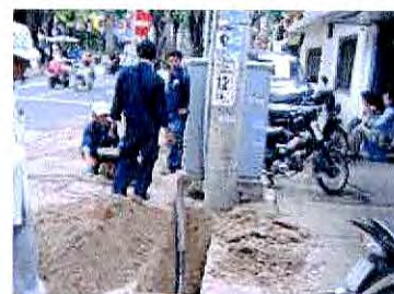
Figure 1. Installation of the main power source
