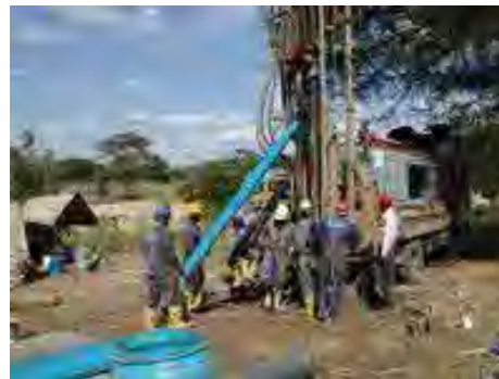
Photo 6-1 Casing Installation
